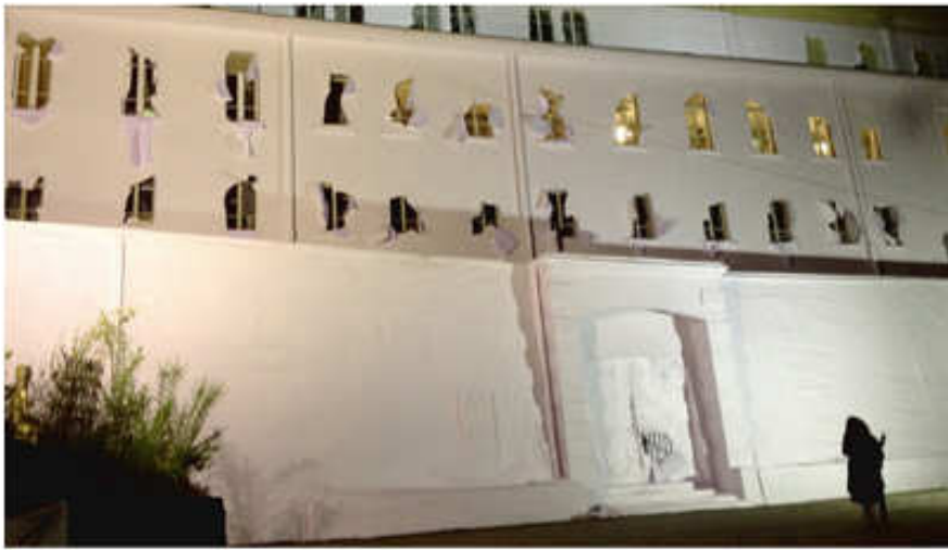
Daniel González, Paper Building , 2016, installation view, photo credits & courtesy Studio Daniel González
